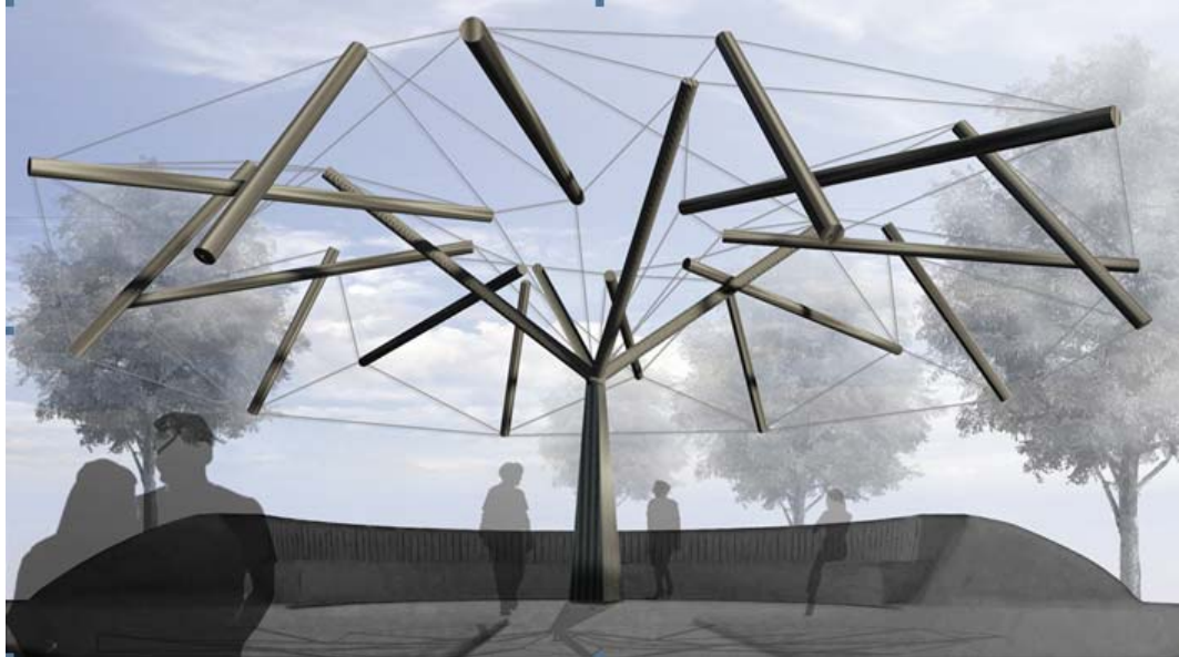
Figure 1: Tensegritree sculpture render. The structure has a height of 7 m, and a diameter of 12 m
