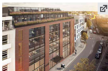
Bewlay House Ben Adams Architects Detailed analysis allowed two lightweight steel storeys to be added without strengthening works. Image: Ink Workshop.
