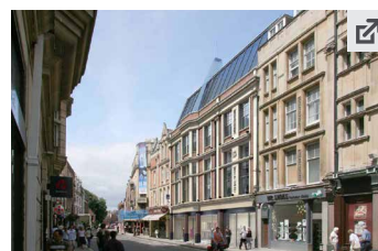
6-12 George St., Oxford Project Orange The reconstruction of a high specification building in a sensitive area behind an historic façade, adding an extra storey in the process. Image: Project Orange.
