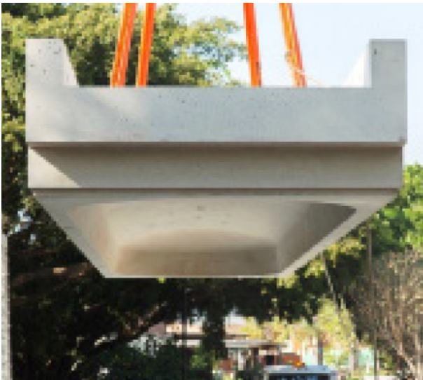
Above: Precast panels at the Global Change Institute made using Wagners EFC
