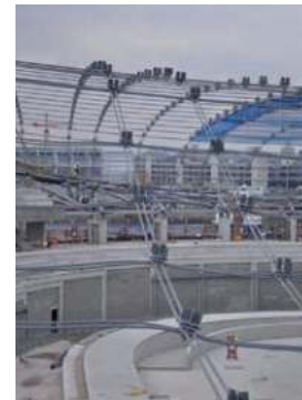
Figure 22 a) Cables laid loose over infield and clamped together at ground level b) Stage 1 of cable lift c) Stage 2 of cable lift – note slack cables in foreground
