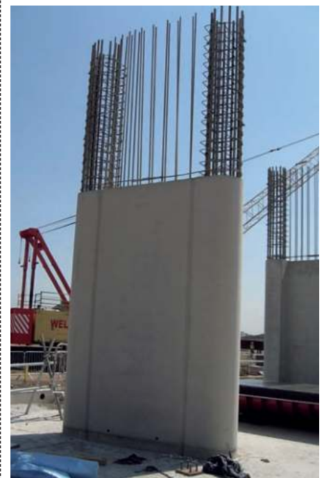
Figure 20 Radial concrete post-tensioned piers
