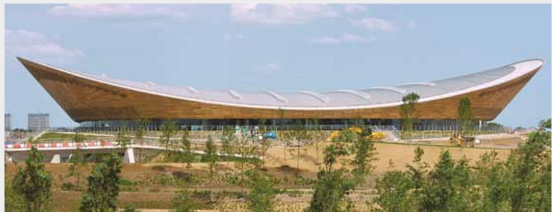
The finished Velodrome has rainwater harvesting and low use fittings that reduce mains water demand by 75%. A total of 5,500 m 2 of Western Red Cedar timber was used for the cladding and 56 km of sustainably sourced Siberian pine timber was used for the cycle track. The structure involved the use of 28% recycled materials (WRAP) and 25% recycled aggregates © ODA
