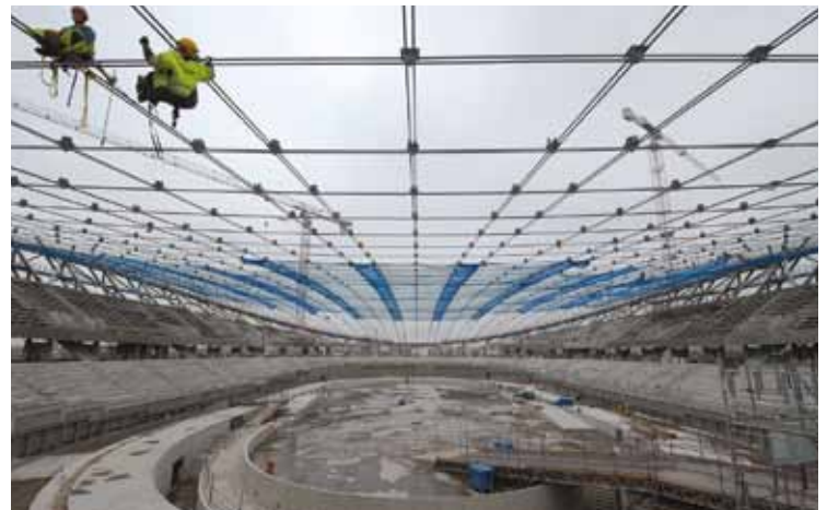
Cables draped over the part-completed arena awaiting lifting and then later during the cable lifting sequence showing the node-connections and cable connections © Expedition
