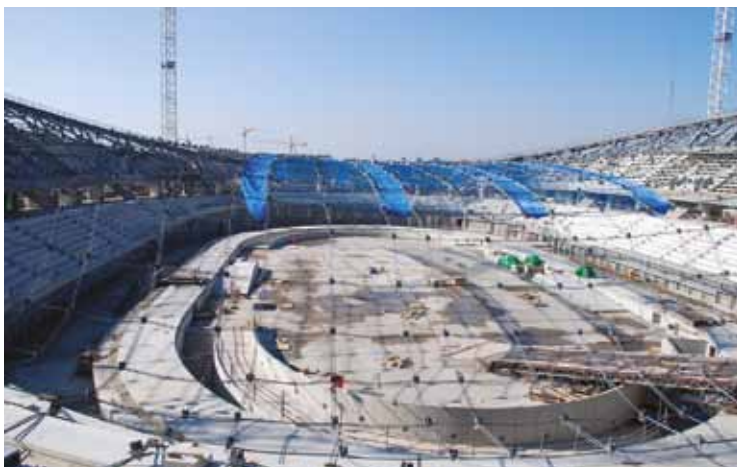
Cables draped over the part-completed arena awaiting lifting and then later during the cable lifting sequence showing the node-connections and cable connections © Expedition
