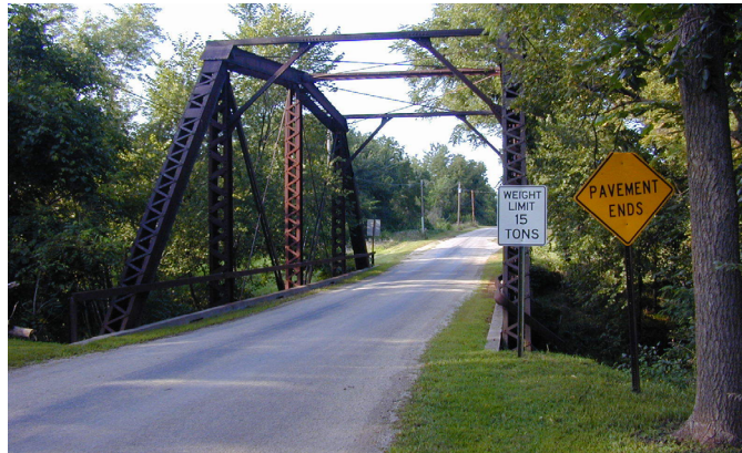
Reclaimed steel/reuse of a span: Duncan Creek Bridge, Kansas, USA. Image copyright Robert Elder. The through truss bridge was constructed in 1935 and, due to the unusual form that does not comply with the codes of the time, it is believed that the bridge was constructed from components from a pre-1900 structure or that sections were relocated and reused.
