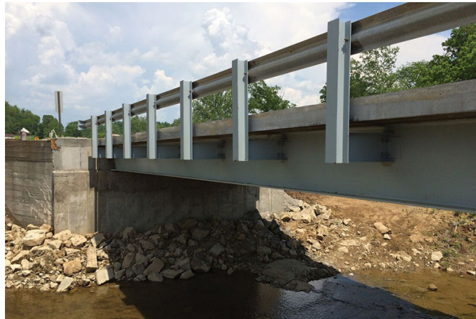
Reclaimed steel: Green Valley road bridge in the United States. Copyright Douglas R. Davis. Steel beams reclaimed from Pleasant Valley road bridge were used to construct the Green Valley road bridge in 2014. A cost saving of $51,000 was reported due to reusing steel in place of new steel. Two other road bridges were constructed using steel from Pleasant Valley, the North Branch and Rural Dale road bridges.
