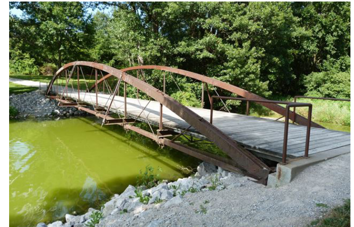
Reuse of span: Dane Road Bridge, Iowa, United States. Copyright Nathan Holth. The original bowstring bridge was constructed in the 1870s before being relocated in the 1990s.
