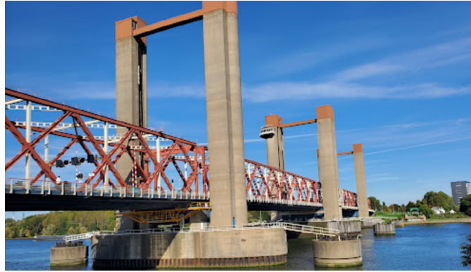
Reuse of a span: Spijkenisse bridge in the Netherlands. Copyright Connie Wang. The remaining four trusses from Moerdijk road bridge were used to construct the Spijkenisse bridge.
