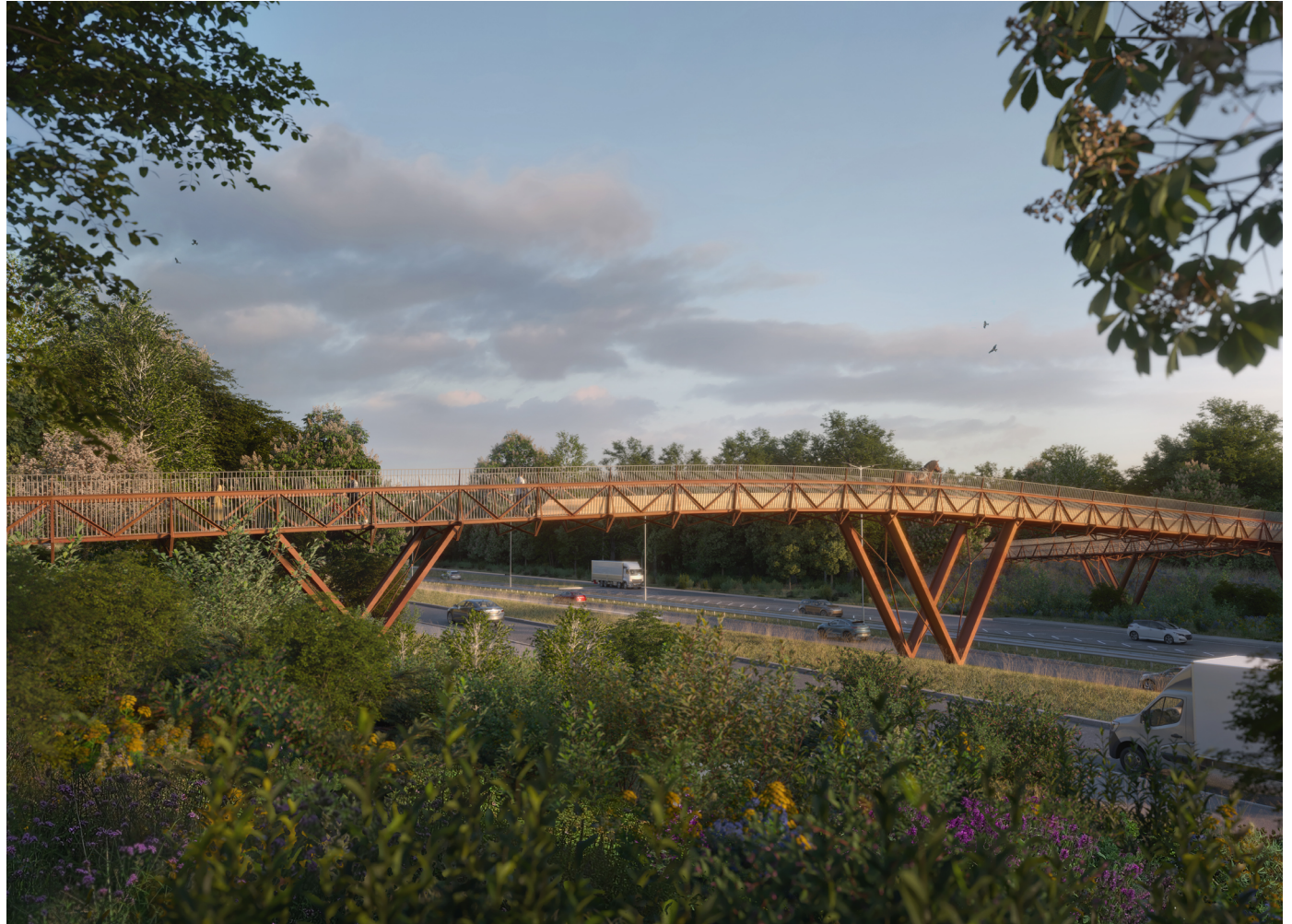
Lower Thames Crossing footbridge competition - shortlisted: Useful Studio and Expedition Engineering. The truss is made of reclaimed steel elements.
