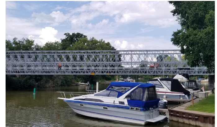
Reuse of a span steel: Image of relocated bridge, courtesy of Acrow. In 2018 the Imperial Road Bridge in Port Bruce Ontario collapsed. Acrow installed a temporary steel bridge. When the new permanent bridge was completed the temporary structure was dismantled, reconfigured and transported to a permanent location 30km away.
