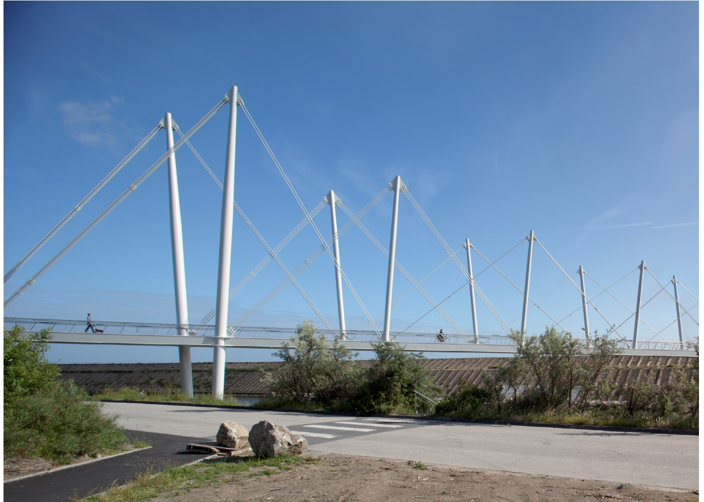
Dunkirk footbridge: the lower part of the masts are of constant sections and could have been designed with repurposed steel. Photo credit: Anne-Claude Barbier.
