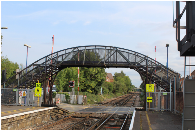
Reclaimed steel: Footbridge South of Wokingham Station. Copyright David Lovell. This 19th-century footbridge is an early example of steel reuse. It is made using reclaimed iron rails.
