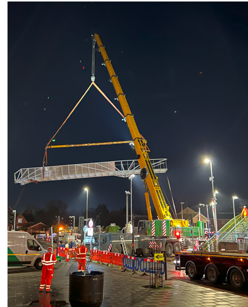
Lifting and positioning of the Tan House footbridge. Copyright Glen Crouch.
