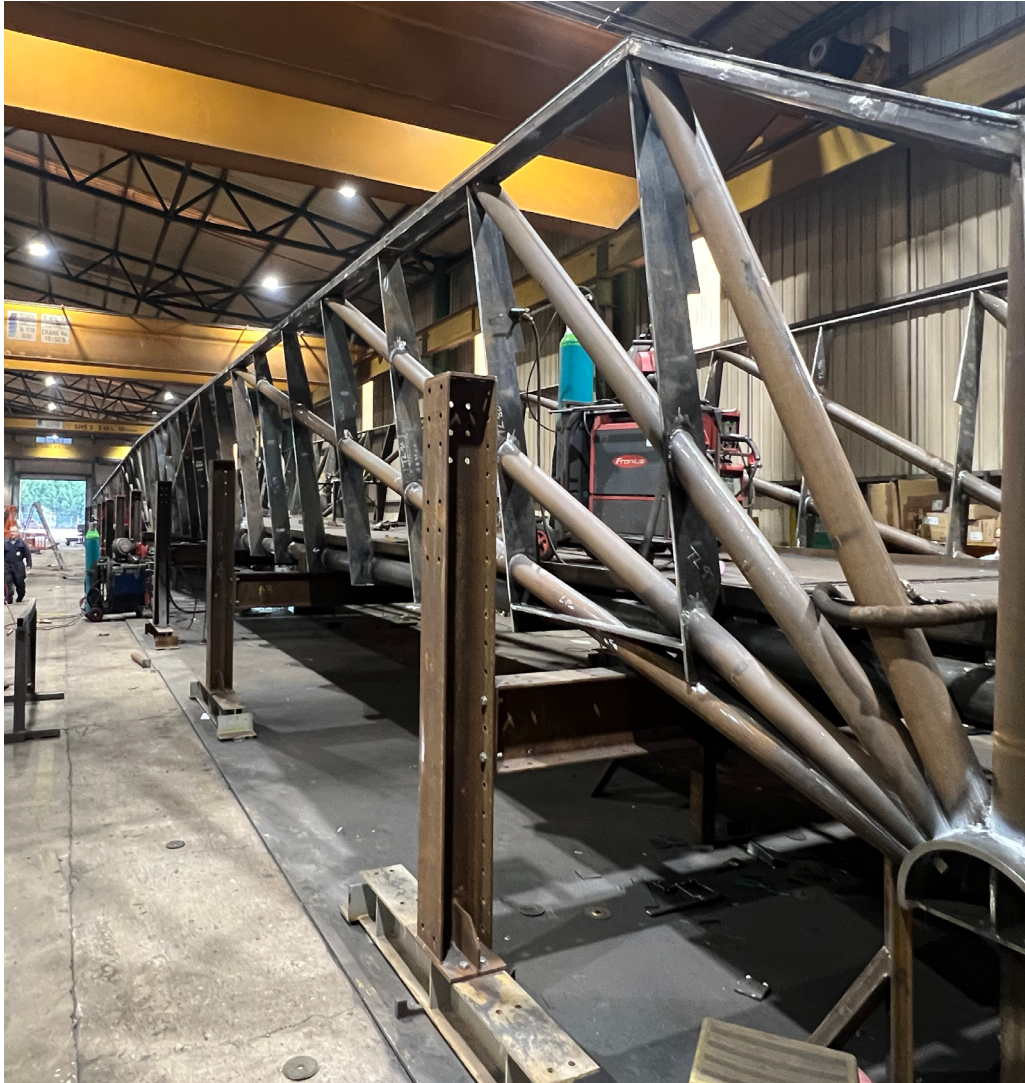
Fabrication of the Tan House footbridge. Copyright Glen Crouch.
