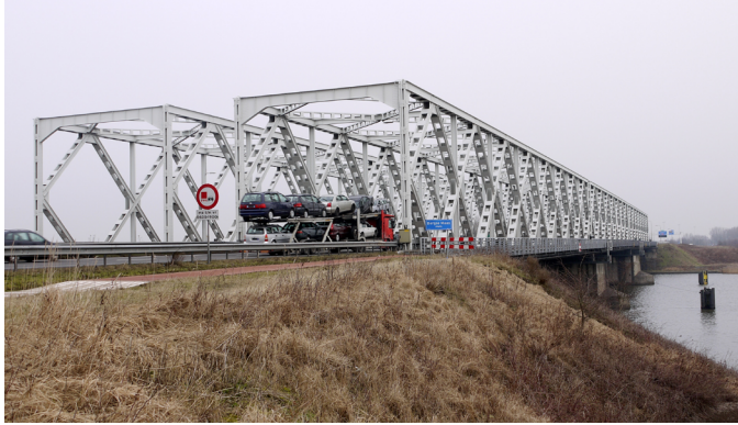
Reuse of a span: Keizersveer bridge in the Netherlands. Copyright CC BY-SA. The Keizersveer road bridge constructed in the late 1970s reused six trusses from the decommissioned Moerdijk road bridge built in the 1930s.
